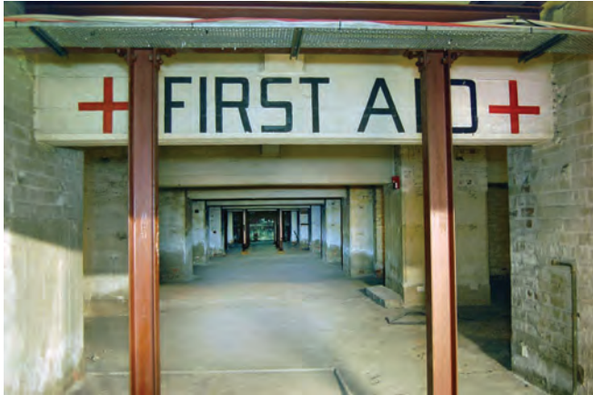
In central Middlesbrough a very large public shelter was formed by joining together a number of shop basements. Although later re-separated, traces remain of its wartime use in signage and localised strengthening with wartime steel struts
